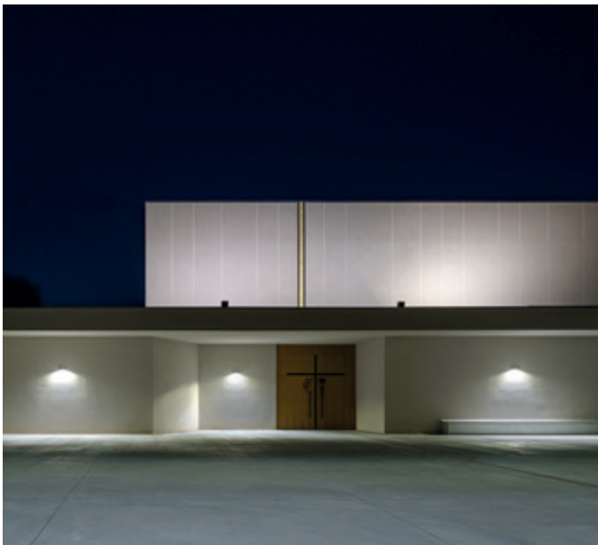
Parish complex - Varignano - Viareggio - Italy
