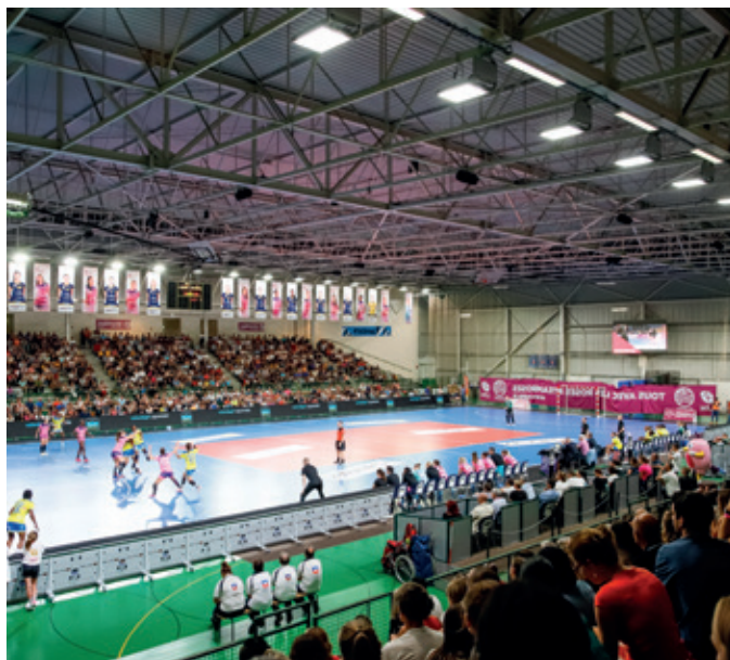
Mangin beaulieu sports complex - Nantes - France
